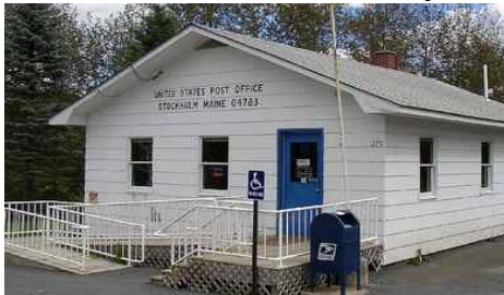
Post Office building in Stockholm, Maine. Note the wheelchair ramp. One must assume most Maine Stockholmers are old.
