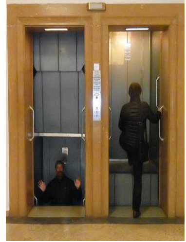
The “pater noster” lift, a vertical conveyor belt.
