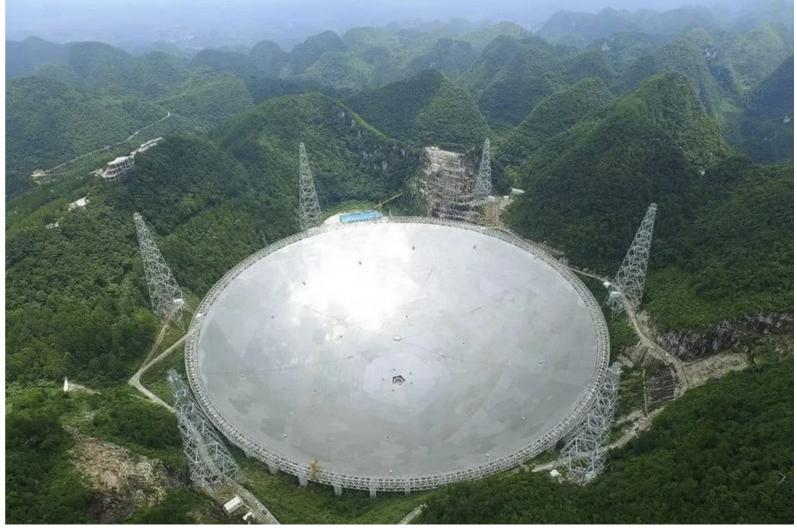
The Spherical Aperture radio Telescope (FAST; Chinese:, nicknamed Tianyan (Sky/Heaven Eye"), is a radio telescope located in the Dawodang depression in southwest China. FAST has a fixed 500m (1,600ft) diameter dish constructed in a natural depression in the landscape. It is the world's largest filled-aperture radio telescope[2] and the second-largest single-dish aperture, after the sparsely-filled RATAN-600 in Russia.
