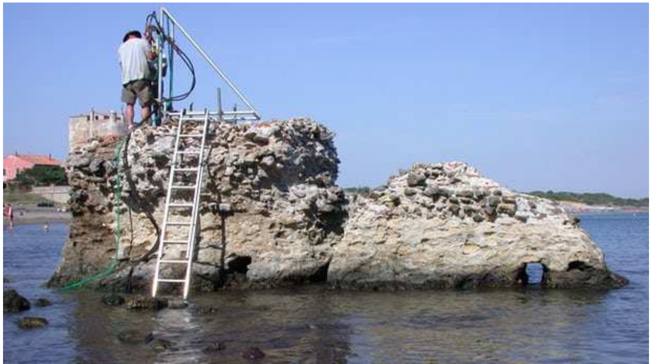
An ancient Roman pier is still standing in a bay in Italy, and researchers have studied samples of the concrete to explore the secrets of its long-lasting strength(Credit: J.P. Oleson)
